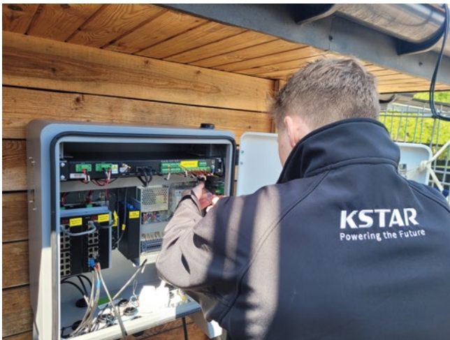
Installers are debugging the product
