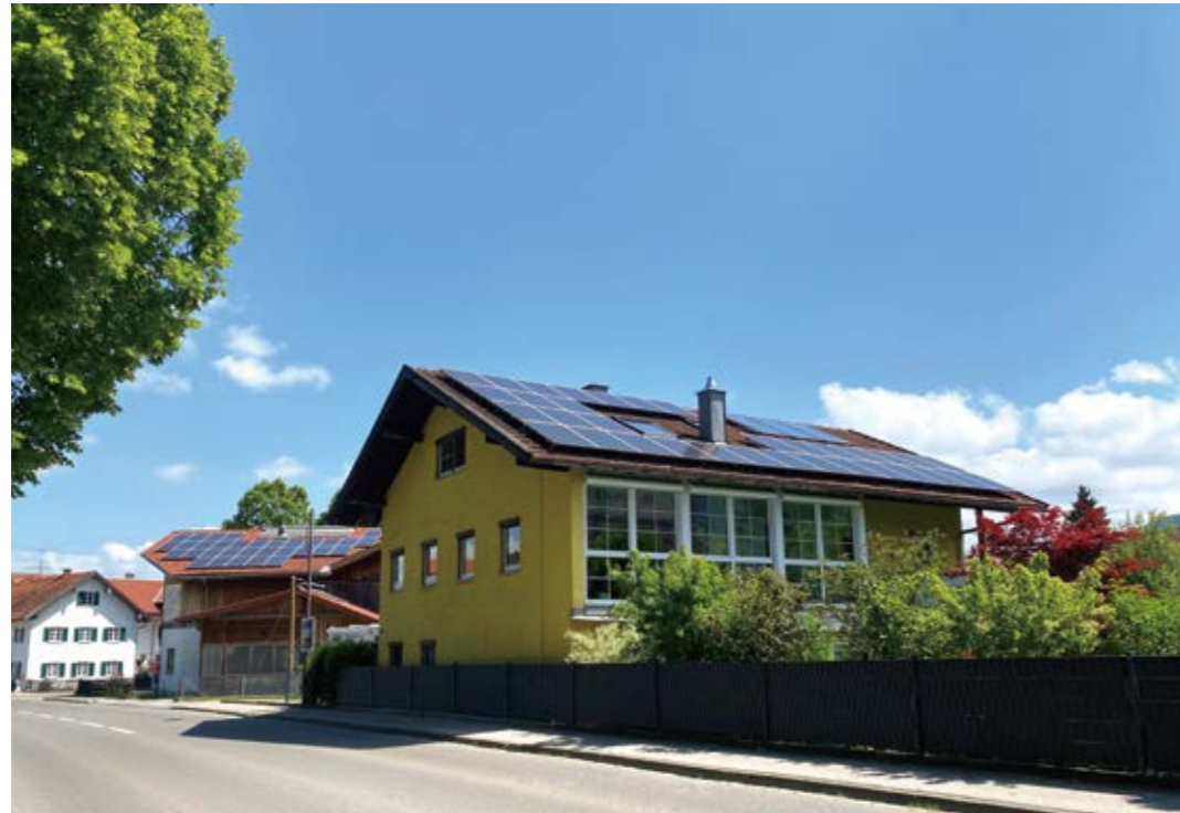
01 Residential ESS Project in Europe
