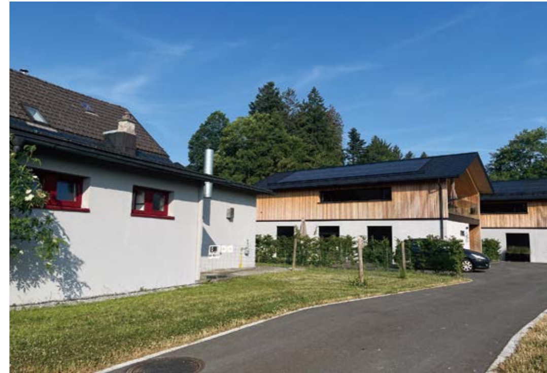
02 Residential ESS Project in Europe
